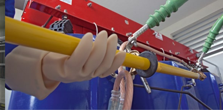
Installation of a Protective Grounding Assembly on a Transformer
