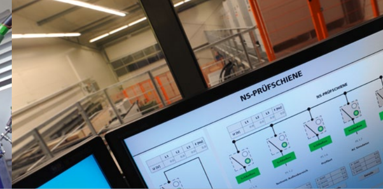
Control Room at PNI Laboratory
